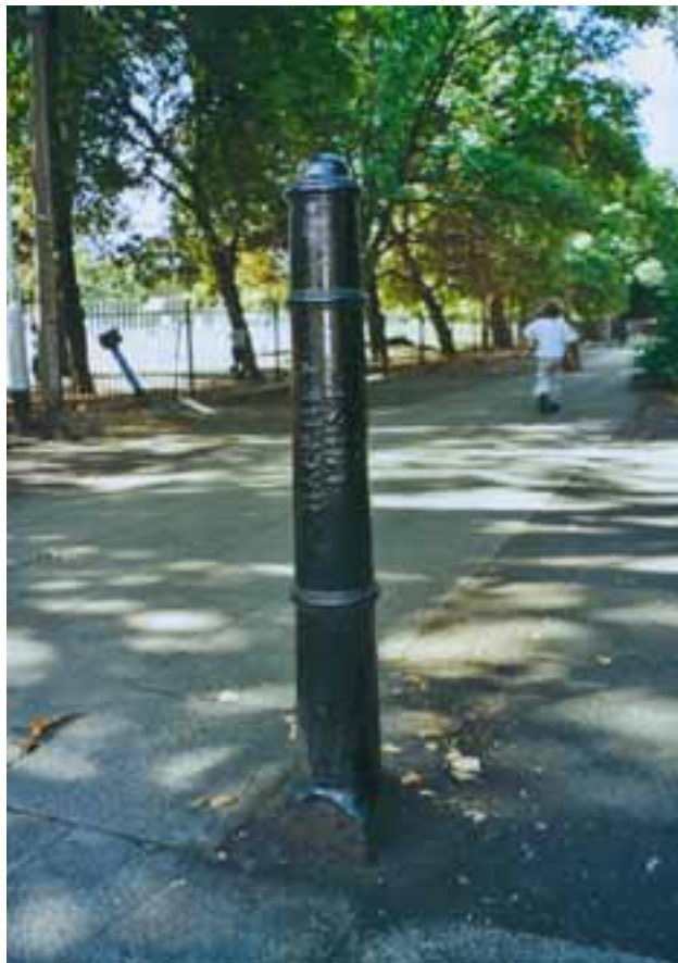
Figure 24 Cast iron bollards in Queen Elizabeth’s Walk
