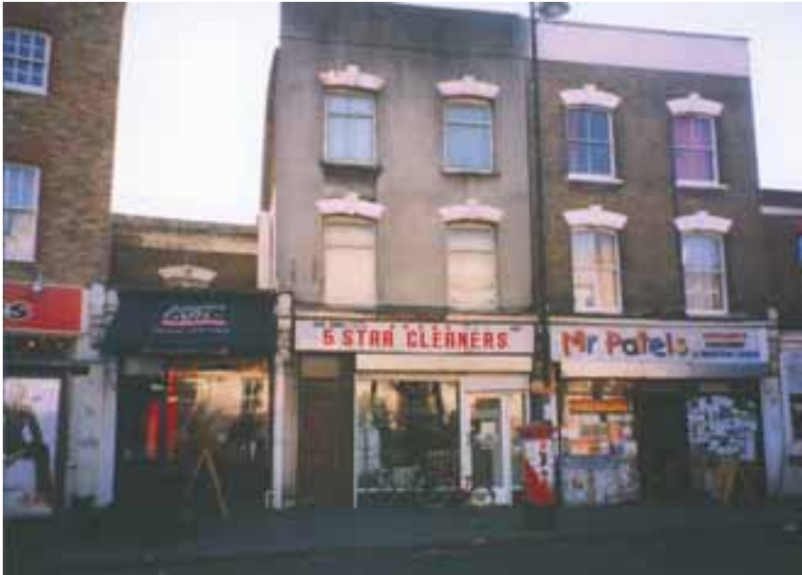
Figure 39 Nos. 189-191 Stoke Newington Church Street
