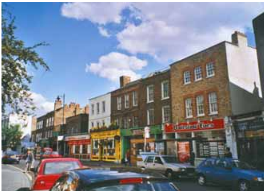
Figure 34 Nos. 177-183 Stoke Newington Church Street
