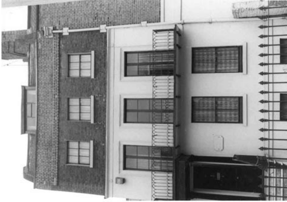
164 Dalston Lane, 18th century, with fine porch of slim columns and fret design on frieze, six panelled door and pointed arch cast iron balcony
