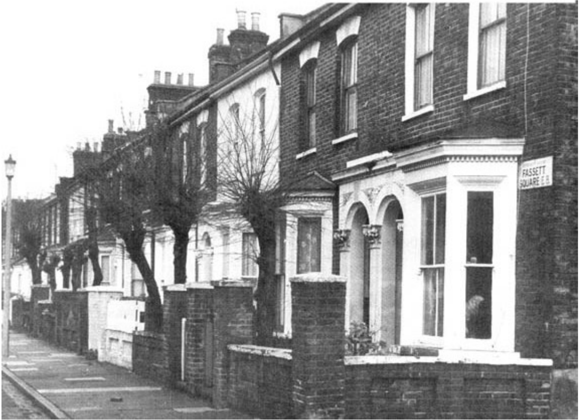
23-38 Fasset Square, early 1860s
