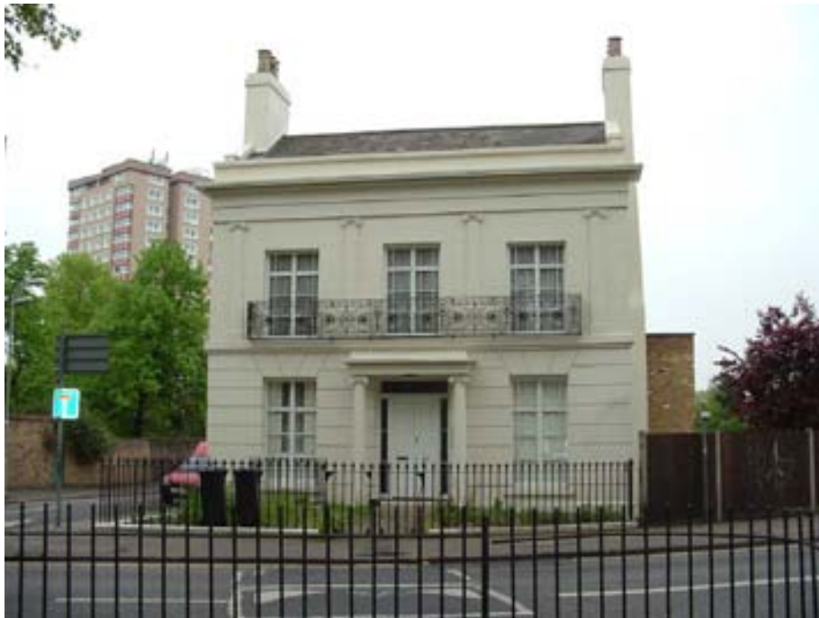
Figure 25: No.170 Lansdowne Drive
