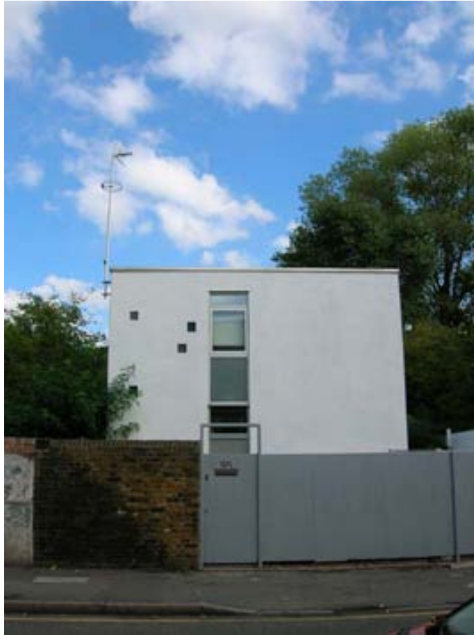
Figure 34: No 95 Landsdowne Drive
