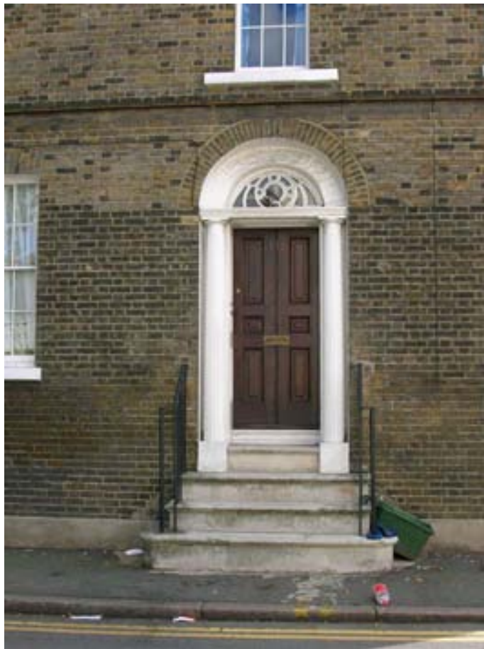
Figure 31: Door at No.172 Landsdowne Drive
