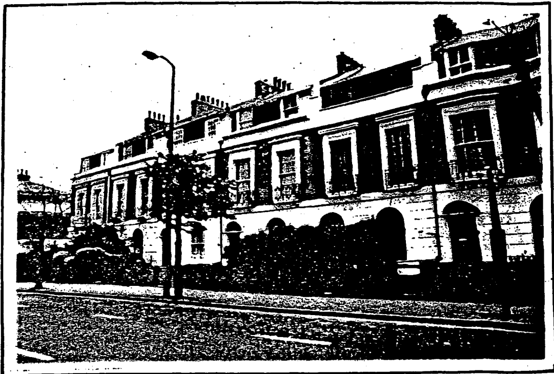
QUEENSBRIDGE ROAD GRADE II GROUP VALUE
