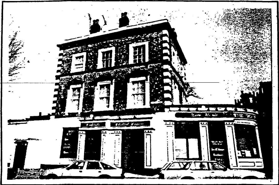
FORMER ALBION PUBLIC HOUSE ALBION ROAD N16 GRADE II
