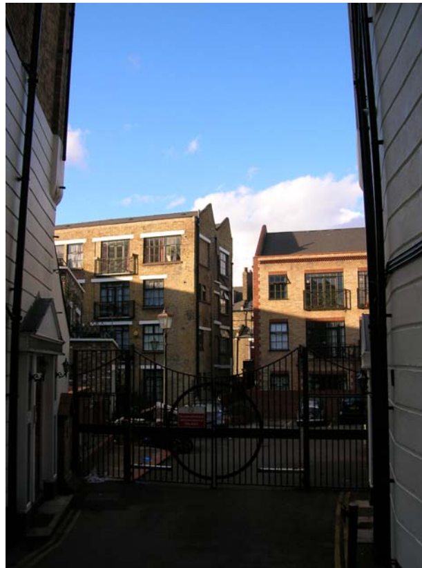
Figure 44: 'Time Square' A sensitive conversion of a former rubber warehouse, plus new build for residential flats to the rear of Colvestone Crescent
