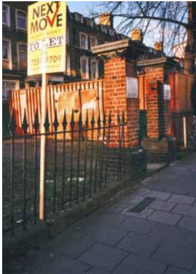
Figure 17 19 th century railings outside no. 1 Stamford Hill
