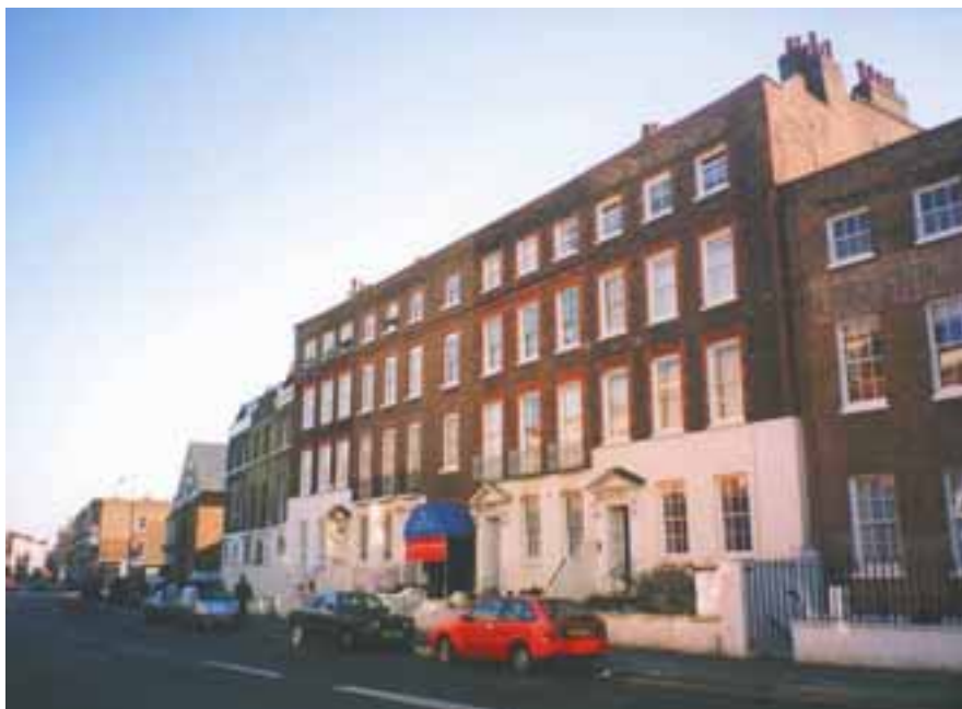
Figure 28 Nos. 75-87 Stoke Newington Church Street
